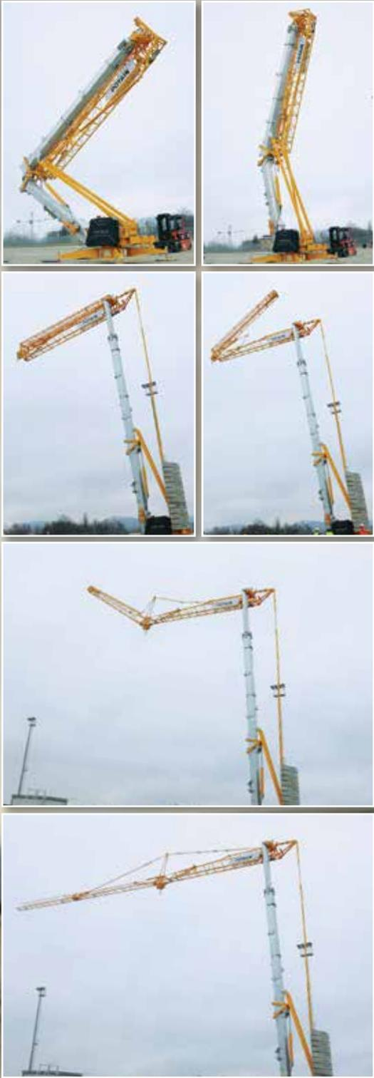
Remote controlled crane erection is quick, convenient and secure.
