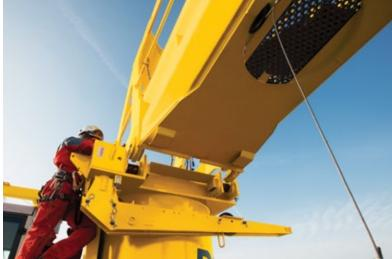
Notches guide and center while connecting counter-jib to mast.
