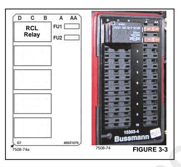
TABLE 3-2: LSI Fuse/Relay Panel, Fuse Identification
