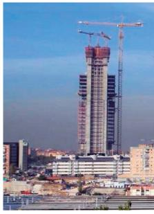
The Spanish company REPSOL ordered one MD 1400 and two MDT 302 for the construction of the «REPSOL TOWER» in Madrid. MD 1400 was erected up to 277,3 m with 7 anchorings and was used to lift 36 t at 38 m radius at 250 m height. Additional 20 t steel structures were installed on the top.
