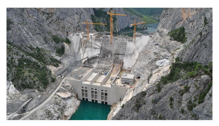
The Boyabat dam project was made with conventional vibrated concrete (CVC), built by blocks using conveyor system and tower cranes. It is located in North Central Turkey near the Black Sea. The main purpose of the tower cranes is to handle 20 t loads such as reinforcement, rebars, conveyor trusses, penstocks and 9 or 6 m<sup>3</sup> of concrete buckets anywhere on the dam project.
