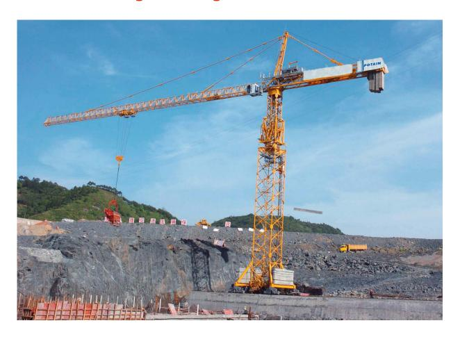
The Qingshuitang Dam is located in the Hunan Province - China, 72 km from Huaihua city. Gezhouba corporation acquired 2 units of MD 1100 (40 t capacity version) for the dam concreting. Both cranes operate with 6 m³ bucket (20 t) up to 52 m radius (jib 70 m) and 3 m³ bucket (10 t) from 52 m to 80 m radius.
