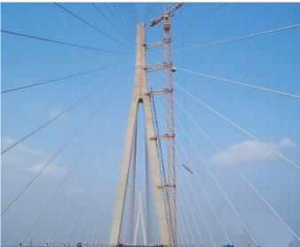
The bridge is located above the Yang Tse river near Nantong. It was constructed with 2 steel and concrete piles reaching 300 m high. The bridge has an overall span of 1200 m. Each pile was built by a MD 3600 tower crane anchored at 6 levels. It was equipped with 2 hoist winches and trolleys: one 20 t trolley for constant loads and one 80 t trolley for heavy loads.
