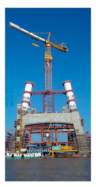
Two giant cranes MD 3600 participated to the construction of the the  $3^{\rm rd}$  Nanjing bridge, located above the Yang Tse River. They were specially designed to lift steel structure elements of 160 t, used for the construction of the bridge piles.
