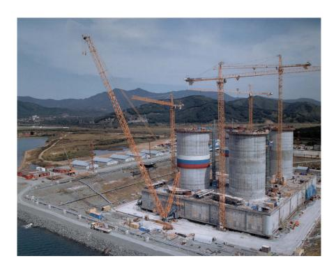
This project consists in the construction of an off shore platform in a drydock near Vladivostok (Eastern Russia). The yard is equipped with 5 cranes: 1 MDT 218 on a travelling chassis, 3 MD 485 B on fixing angles and 1 MD 485 B on chassis.
