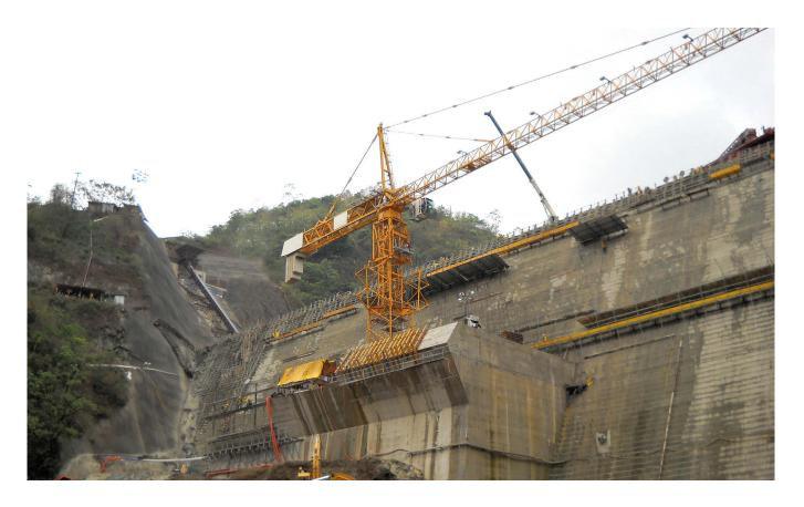
Pirris is one of the largest dams ever built in Costa Rica. ICE company purchased a new MD 1100 to build the dam. The crane has been chosen for its outstanding performance and its compactness for transportation. Considering the seismic constraints of the jobsite location, the crane was reinforced to withstand maximum accelerations of 0,16 g.
