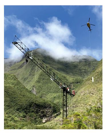
After manufacturing, the crane was shipped to the GLI yard on La Réunion, where the erection team practiced assembling and disassembling prior to installing it, to be sure of the weight, slinging points and work plan.
