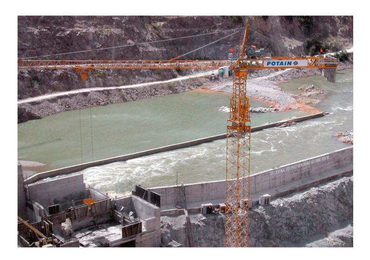
The Vietnamese Son Da Corporation company ordered 4 MD 900 B cranes for dam construction. The 250 LCC hoisting mechanism enables a productivity of approx. 70-80 m³/h depending on the site conditions. Trolleying and slewing mechanisms with frequency variations.
