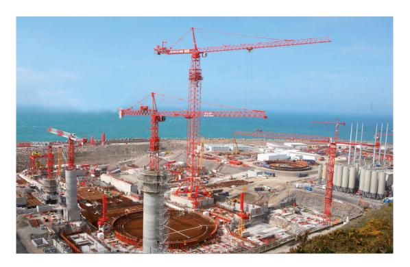
Bouygues company purchased an MD 3200 to build the EPR nuclear power plant in Flamanville. The liner was made of 40 t curved steel plates welded on-site. Other general equipment were lifted by the crane. The MD 3200 overflew the fleet of various types of tower cranes, mainly Topless, all calculated in accordance with the strong wind specifications of the French northwest coast (more than 200 km/h) as well as the proximity of the cliff.
